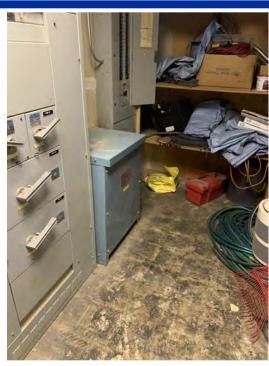
Photo 22 Northern electrical room with dry-type transformer.
