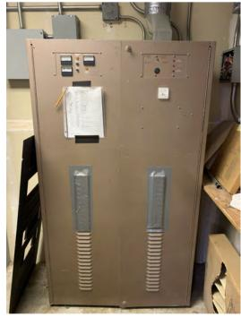
**Photo 21** School backup power equipment. Formerly contained batteries
