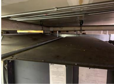
**Photo 24** Ducting and fiberglass insulated water lines in equipment loft
