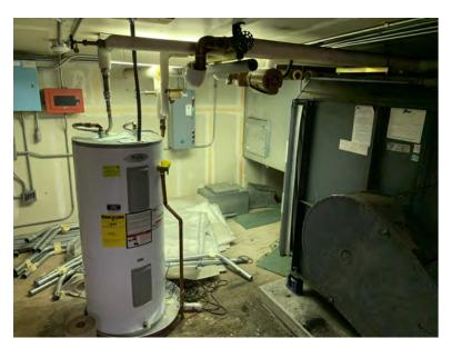
**Photo 23** Water heater and fiberglass insulated water lines in equipment loft area above custodian room
