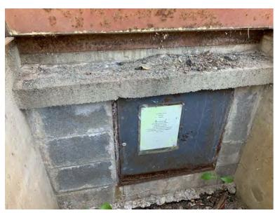
Photo 14 Entrance to pipe chase beneath northern half of northern building wing. Signs warn of presence of asbestos
